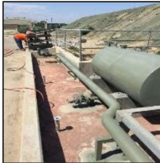
Priming of piping and tanks
