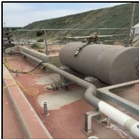
Sandblasted to bare metal
